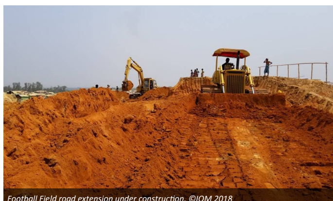
Football Field road extension under construction. ©IOM 2018
