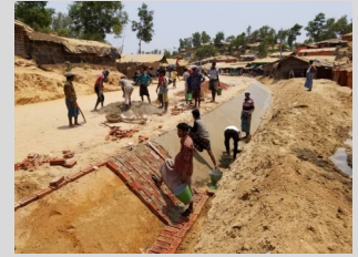
Construction of drain on Pan Bazar Extension Road.
