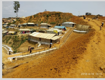
Access up and over the Army Road - connecting Camp 10 to Camp 18.
