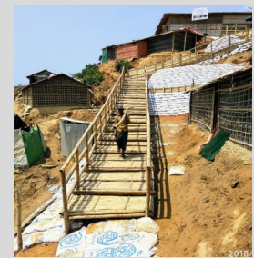
Elevated bamboo steps leading to IOM Health Clinic.
