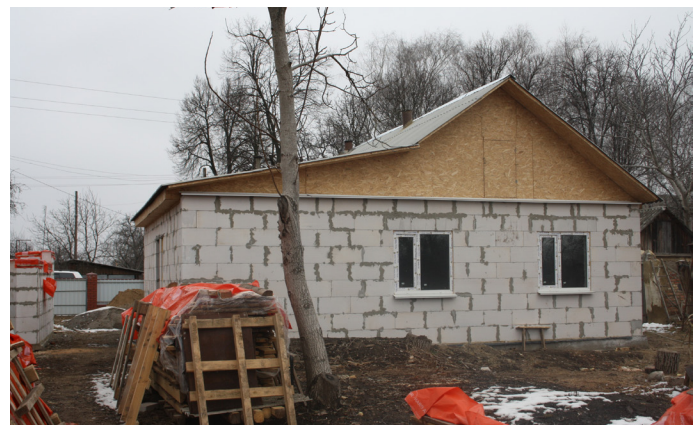
New home of Borys needs to be completely renovated
