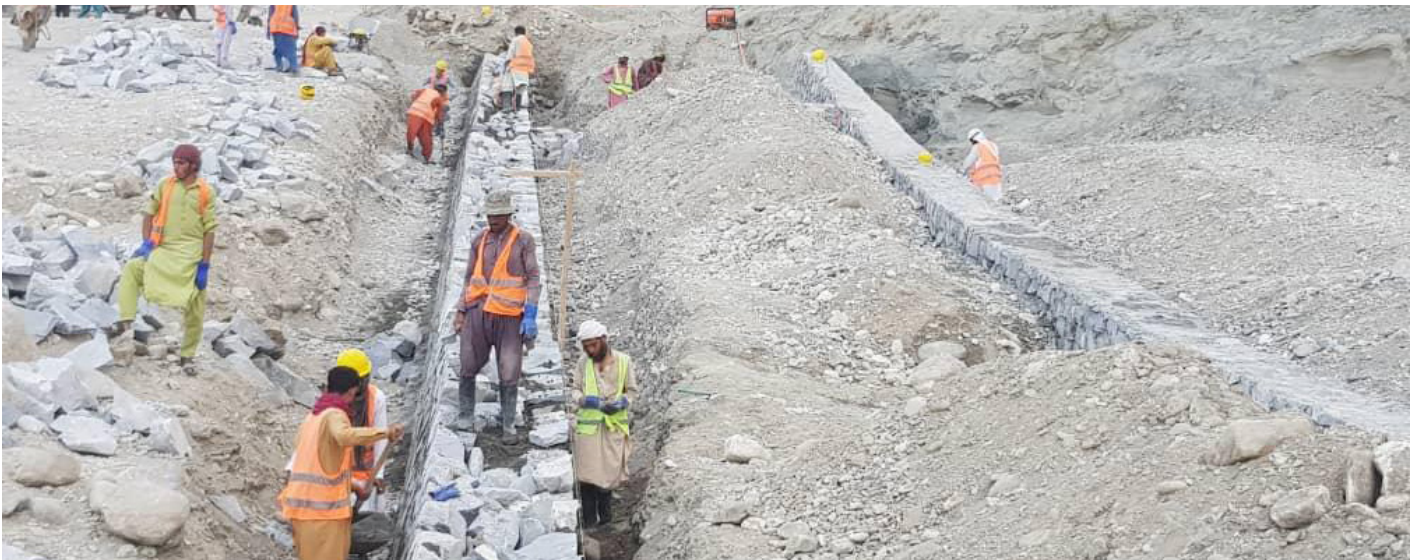
Construction of causeway (disaster and risk mitigation infrastructure) in Nangarhar ©IOM 2021
