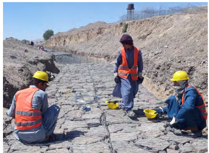
Construction of a gabion wall to reduce disaster risks in the village of Doghni Qanat Wakil, Herat province
