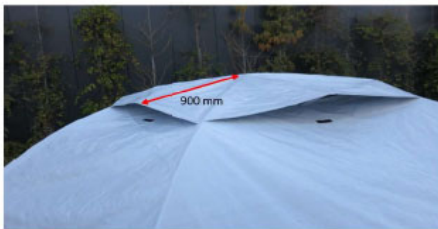
Picture 37 Top vents is located at 900mm from the roof centre
