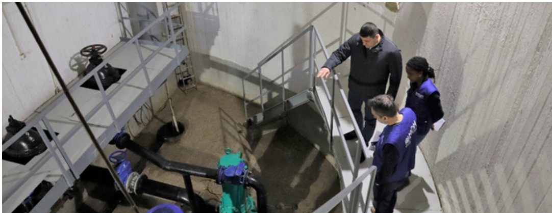
Replacing old pumps and equipment , Ukraine © IOM 2022
