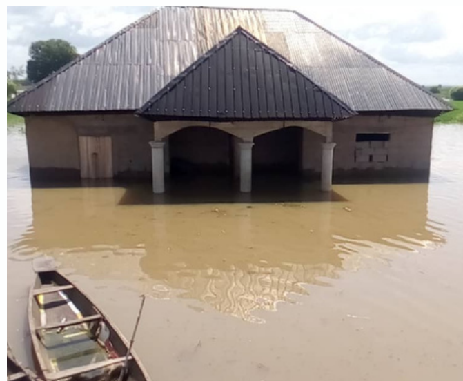
Affected flooding area Maiduguri- Nigeria © IOM 2022
