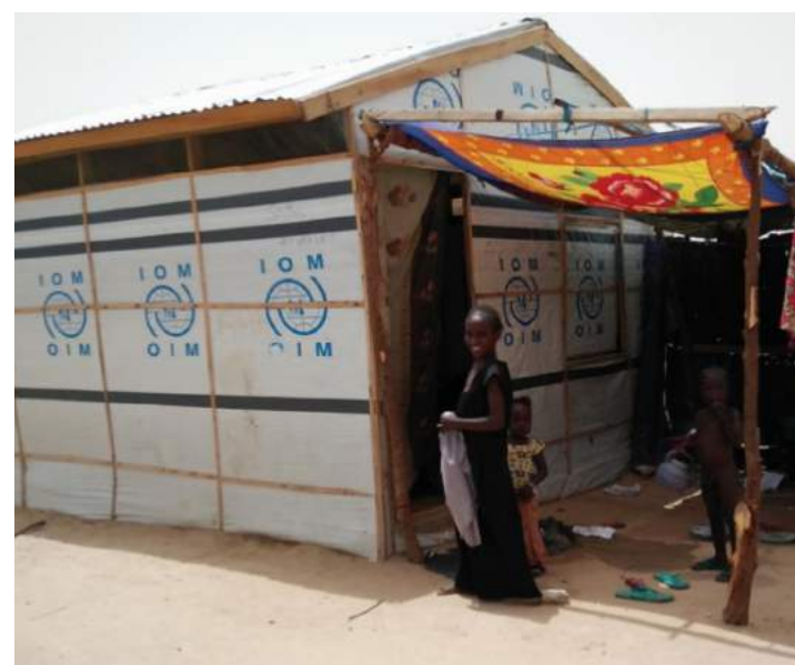
Transitional shelter, Bakasi Camp, Borno State, Nigeria © IOM Nigeria 2017
