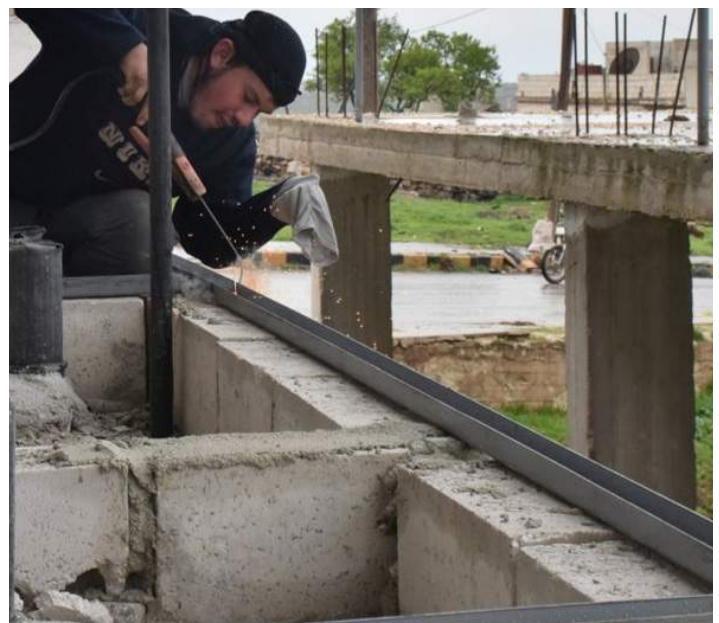
Contractor working on housing rehabilitation, Syria, © IOM 2017
