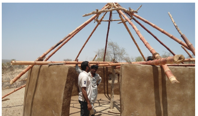
Early Recovery Shelter under construction in Sindh © IOM 2012
